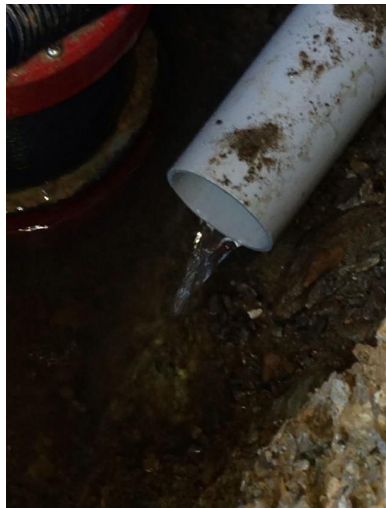
The slab immediately after pouring. Note the discharge pipe (arrow) exiting from under the slab.
