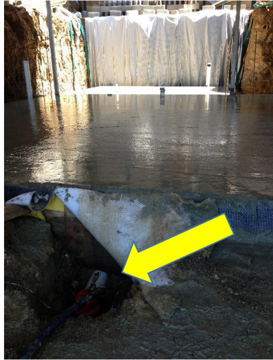
The slab immediately after pouring. Note the discharge pipe (arrow) exiting from under the slab.
