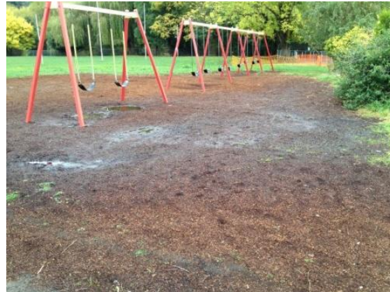
Figure 2. Playground with persistent flooding.
