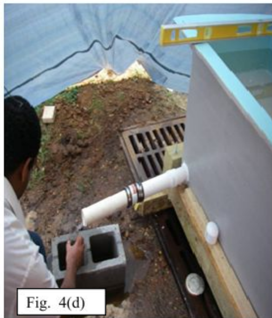
Figure4. Capiphon™ installations procedures in a fiberglass trough 3m long and 0.6 x 0.6m in cross section.
